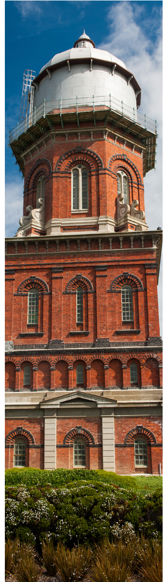
Water Tower, Invercargill
